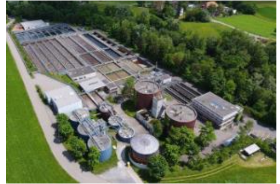
Wastewater treatment plant Schönau
